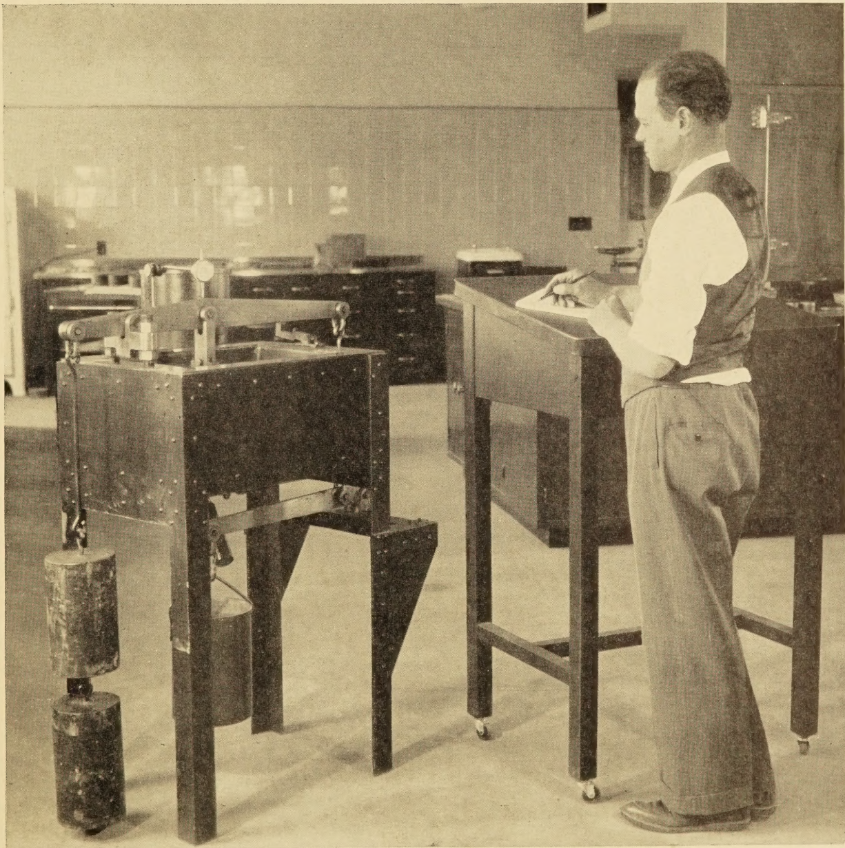
PERFORMING BENDING TESTS ON BITUMINOUS MIXTURES
